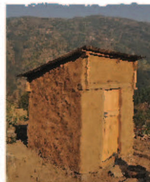
One of many completed toilets in Rakha.
