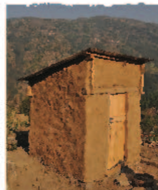
One of many completed toilets in Rakha.
