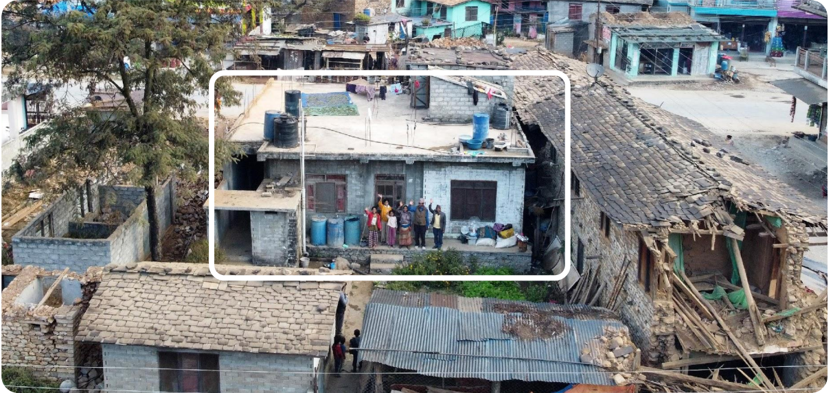
✓ CSEB single-storey with RCC frame & slab roof. Bhrei 01, Jajarkot
