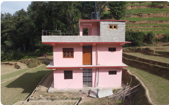
✓ 2.5-storey RCC and CSEB, Tribeni, Rukum West
