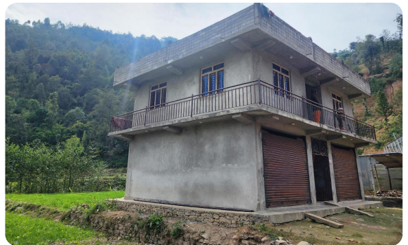
✓ 2-storey RCC and CSEB Tribeni, Rukum West
